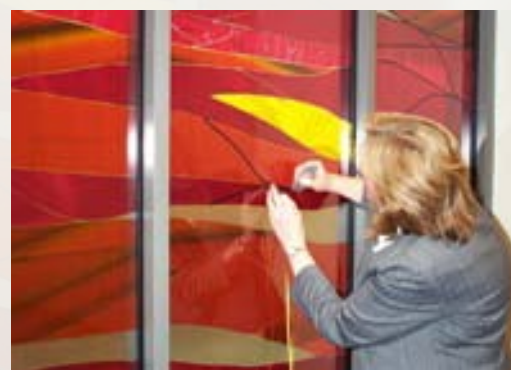
Myrand installs the special materials used to mimic the lead caning that appears in traditional stained glass windows.
