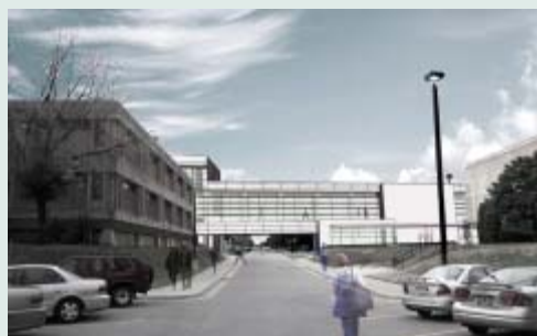
A view of the walkway that will connect the Shiffman Library and the Medical Education Commons to Scott Hall.
